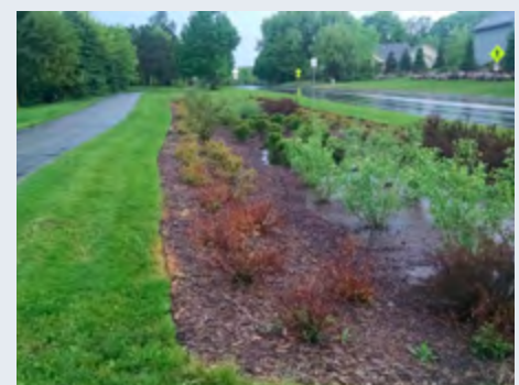
This roadside rain garden along Interlachen Parkway was installed as part of the 2016 Roadway Rehabilitation Project.
