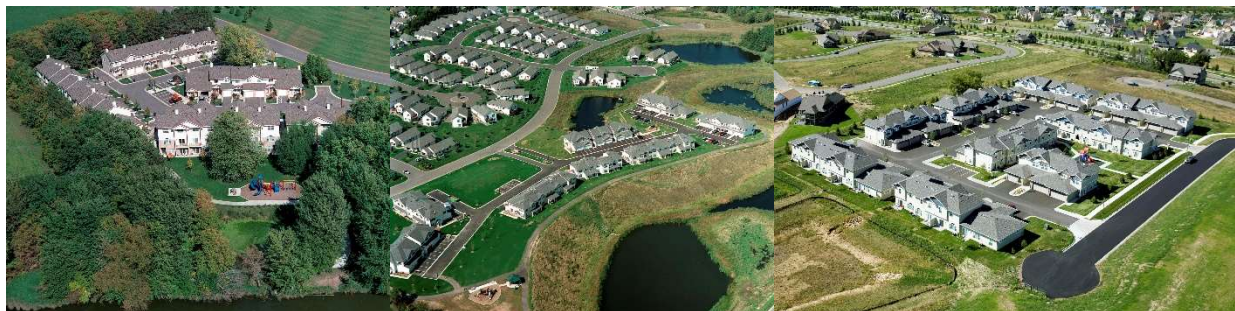
These three rental townhome developments in Woodbury offer examples of affordable rental communities developed using the federal low income housing tax credit tool.
